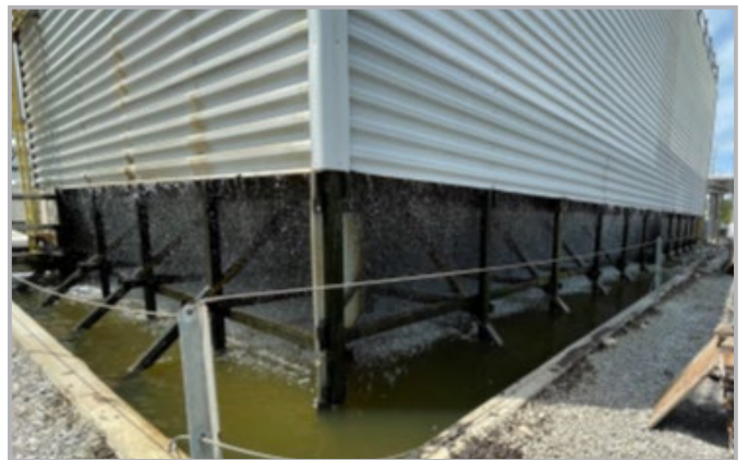
Back corner of the cooling tower basin two months into the trial. The water fall and wind circulation improved after SurfClean 2.0 application, indicating cleaning of the cooling tower fill.
