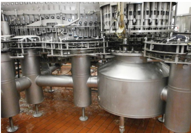
After FillerScrub™ Application
