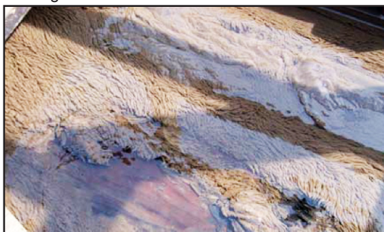
Cooling Tower Deck BEFORE CL206 Addition
