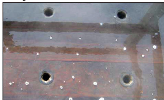
Cooling Tower Deck AFTER CL206 Addition
