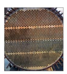
This ammonia precondenser on the urea cooling tower loop shows no evidence of deposition, fouling, or corrosion after 1.5 years on the FlexPro program.
