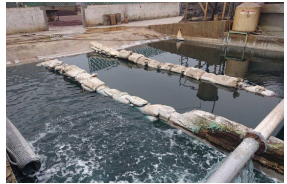
AFTER: Low turbidity in the settling ponds
