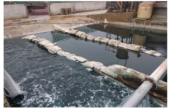
AFTER: Low turbidity in the settling ponds
