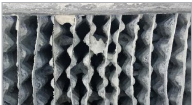
Cooling tower fill with major scaling issues before CL5660 cleaner was applied.
