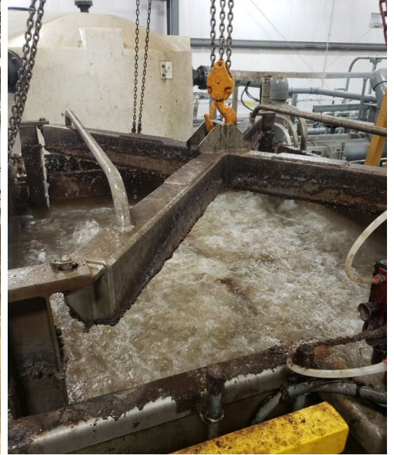
AFTER: FO180 application reduced foaming significantly
