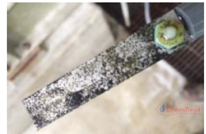
Elevated pitting corrosion in the untreated circuit.
